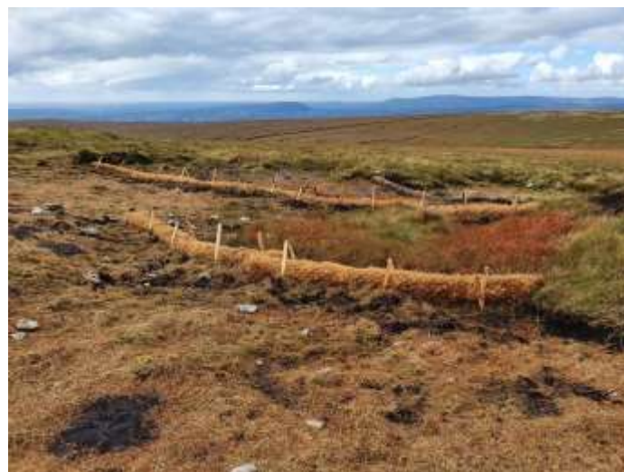
New timber dams installed in the narrow gullies and new coir logs in place on the summit: both will slow the flow
